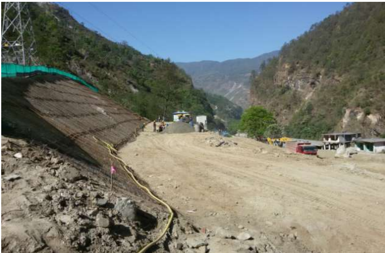
Headworks-Desander- slope excavation above Araniko Highway
