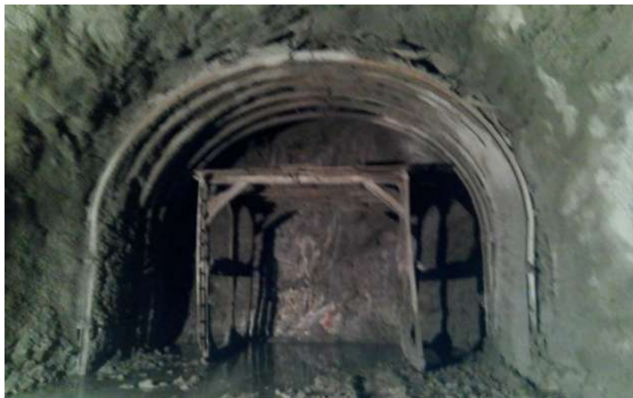
Adit 2 via HRT
