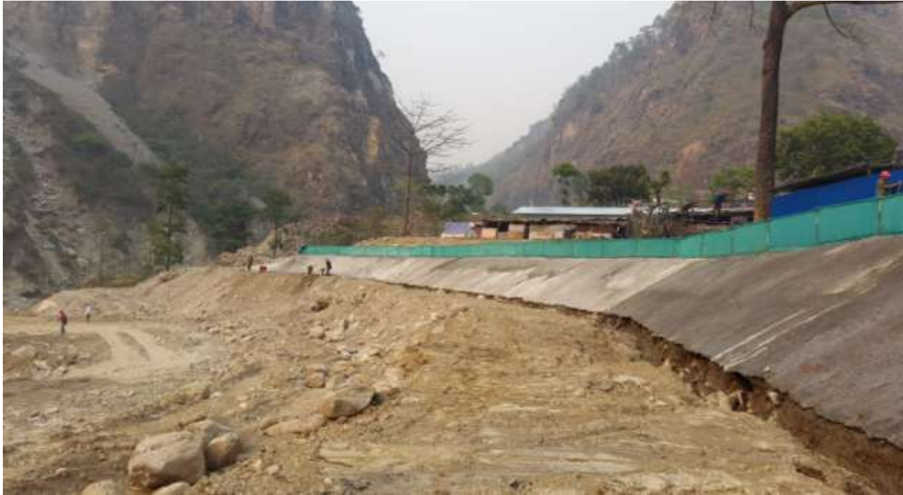
Headworks left bank slope excavation below Araniko Highway
