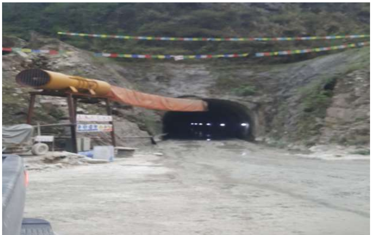
HRT Inlet Tunnel
