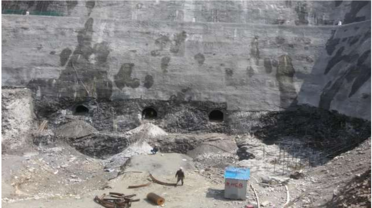
Power house excavation completed and Manifold tunnel excavation in progress
