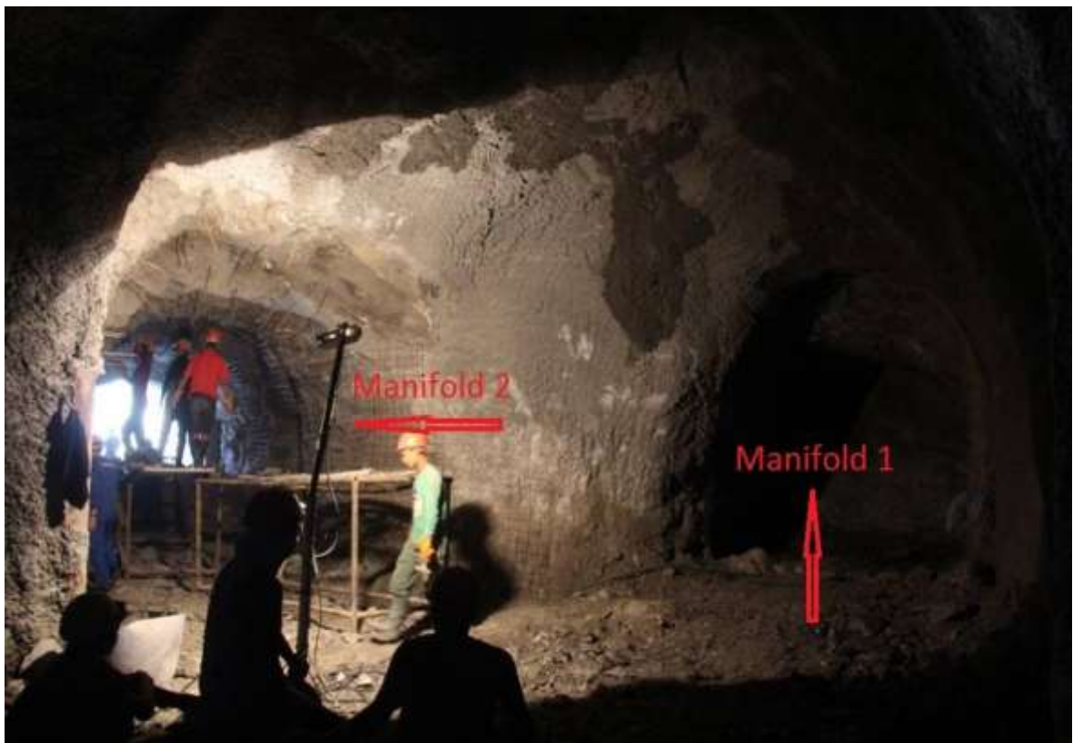
Breakthrough of three manifold completed
