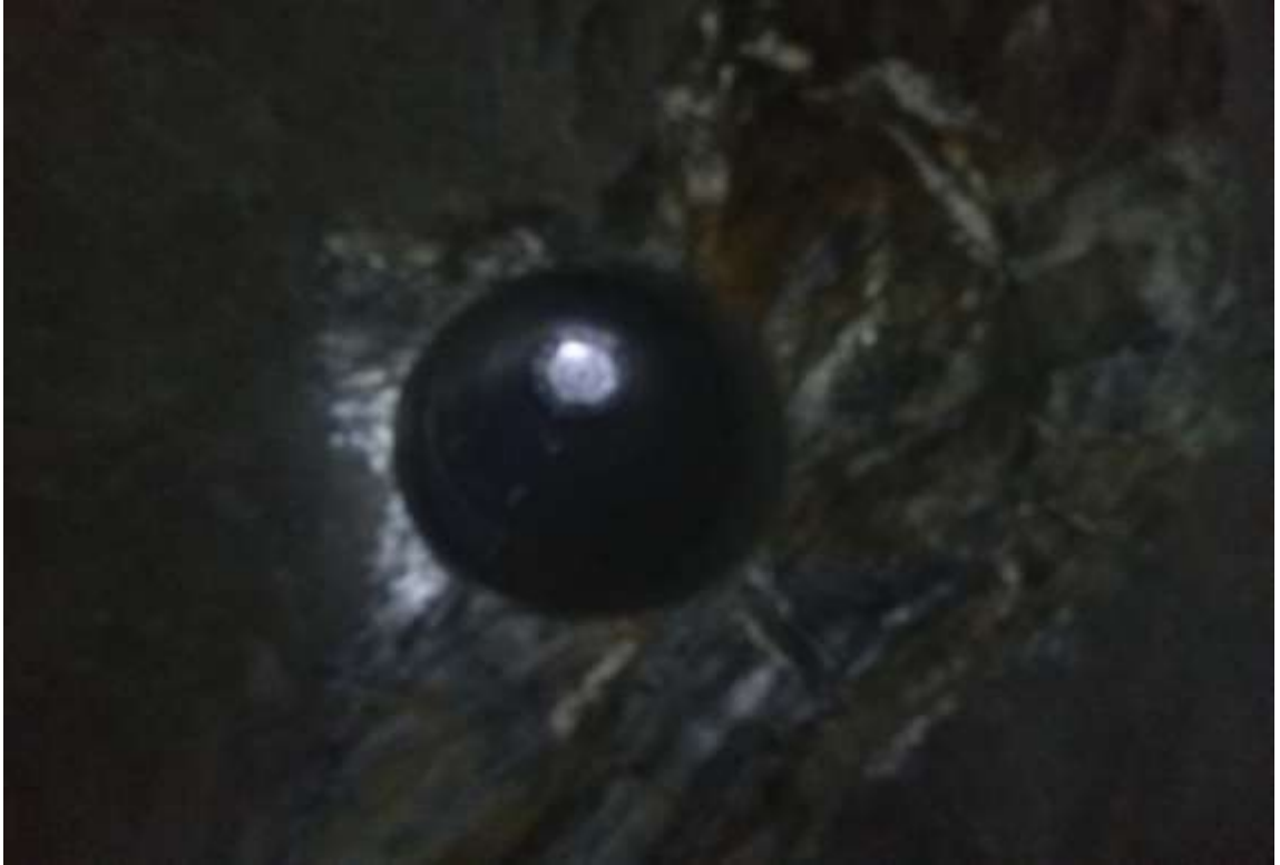
Surge shaft -Pilot hole at HRT
