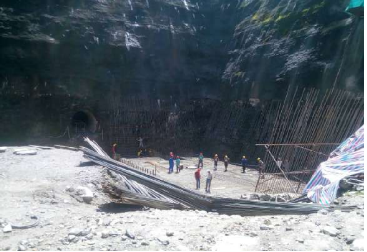
Preparation of concrete in auxillary bay in Powerhouse
