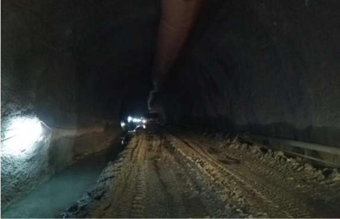
Adit 1 Via HRT
