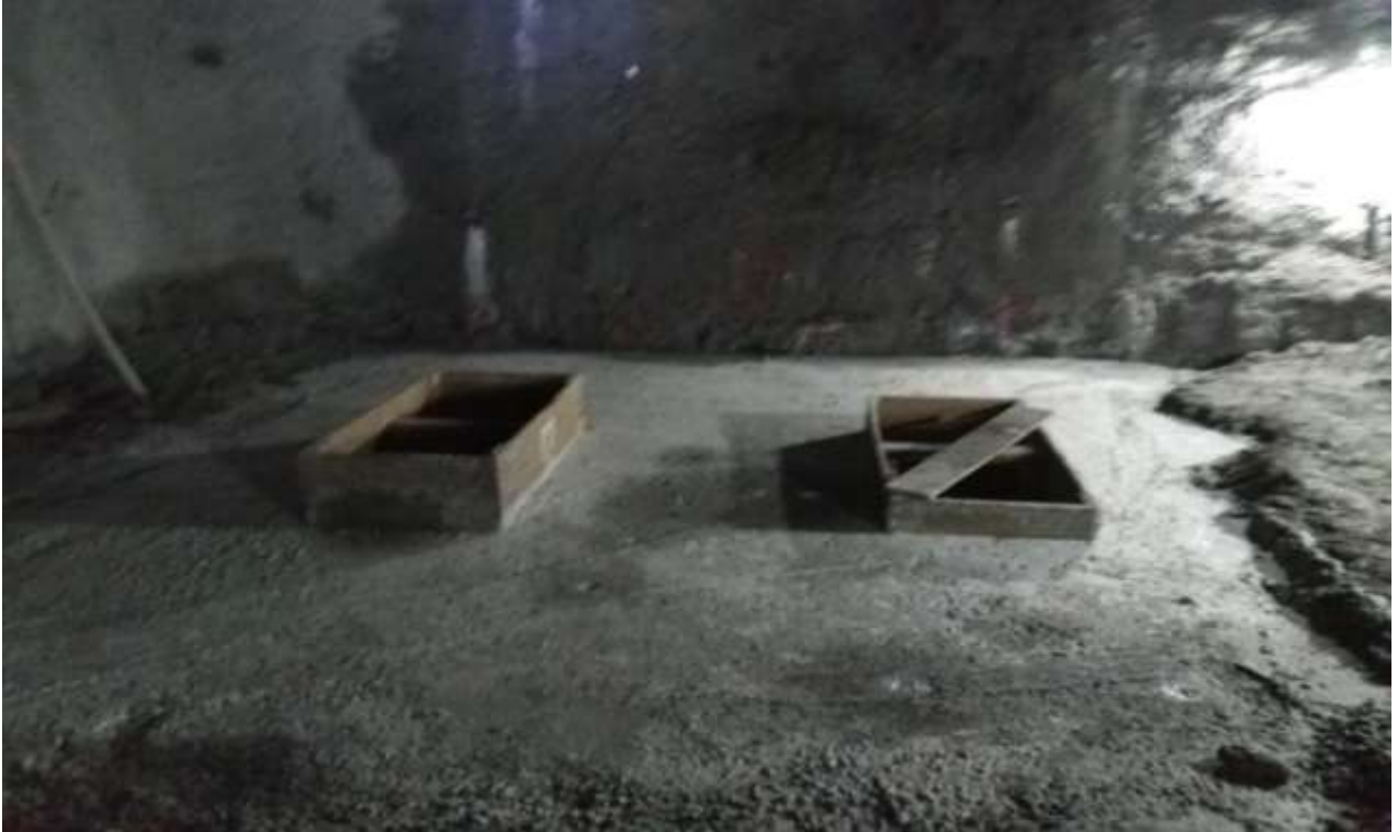
Surface preparation for Vertical shaft
