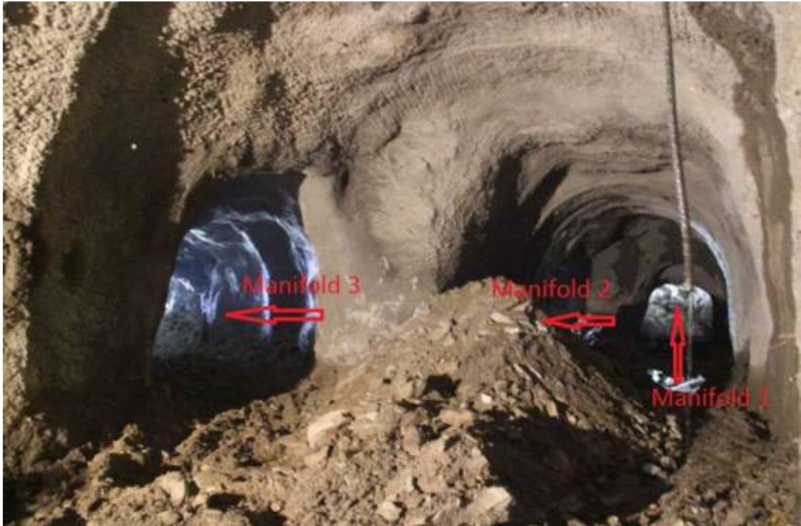
Breakthrough of three manifold completed
