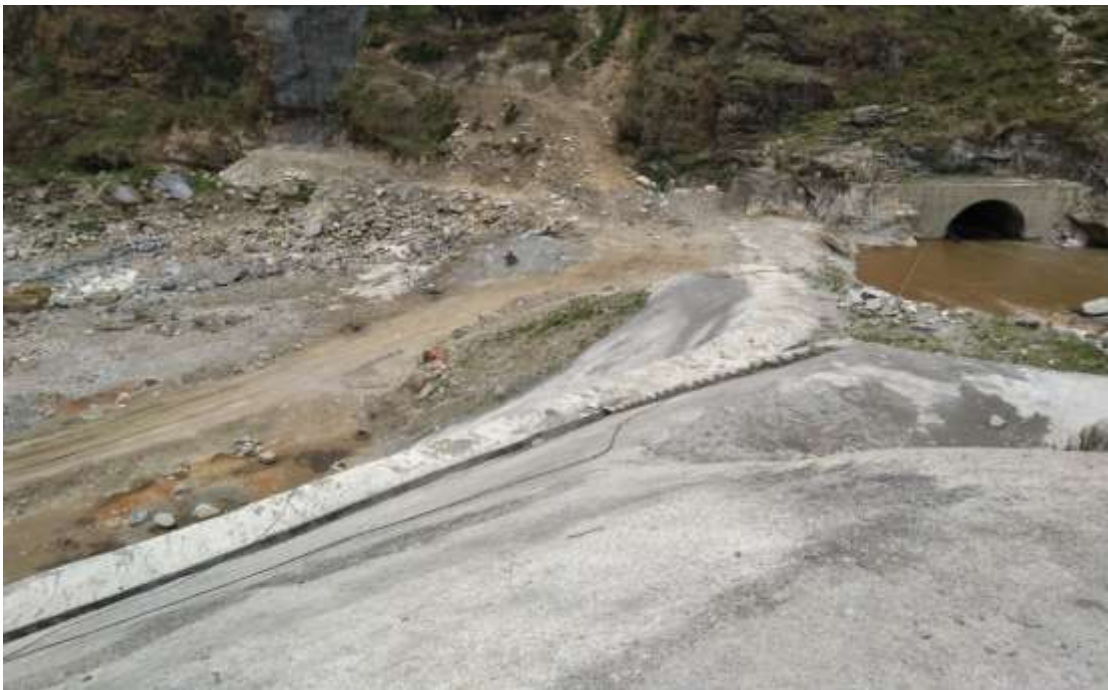
Headworks :Drilling and Jet grouting works of u/s coffer dam completed
