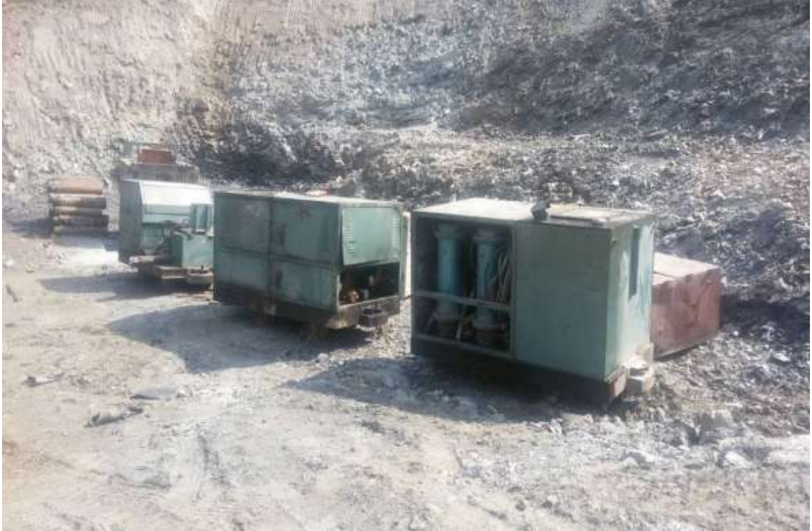
Raise Boring Machine at Surge tank
