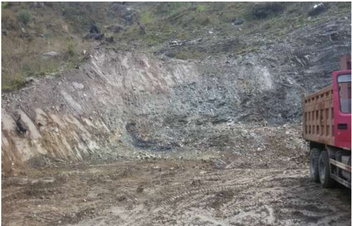
Surge Tank excavation
