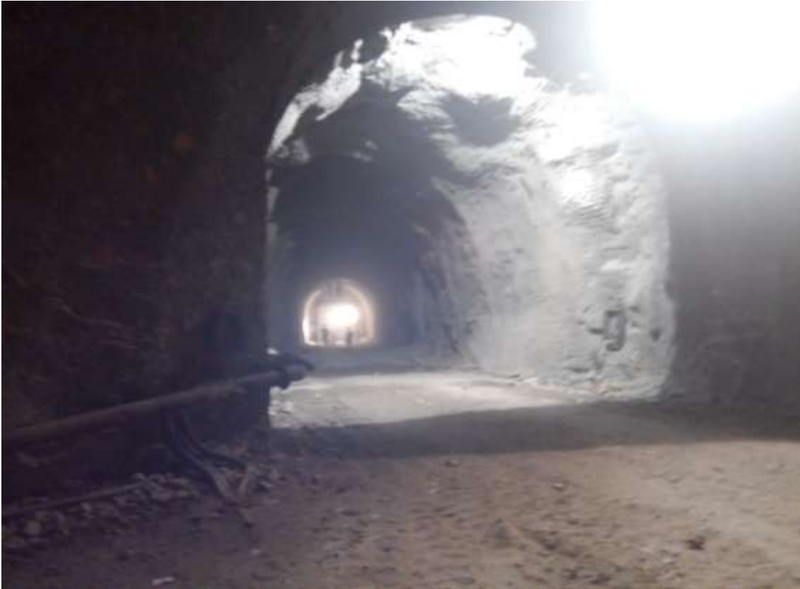
HRT From Adit-1
