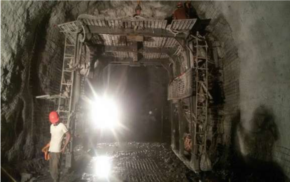
Penstock From Adit-2
