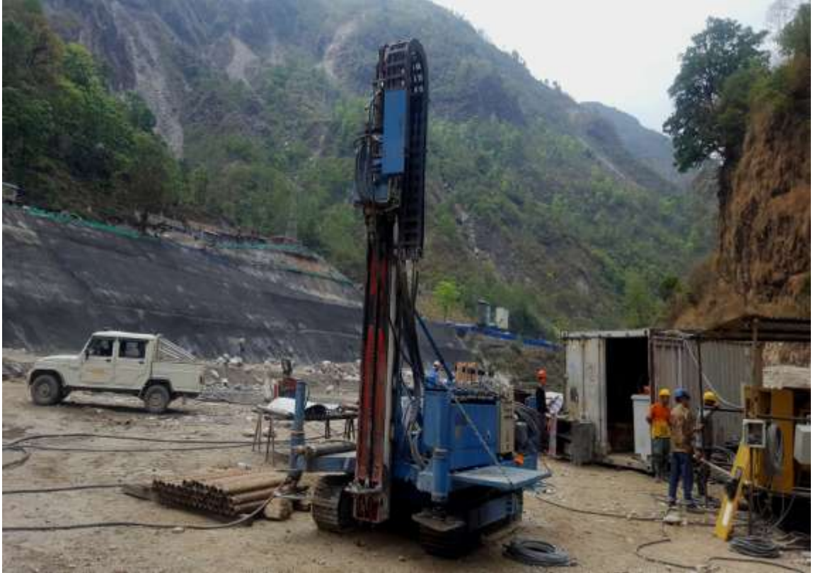
Headwork-Grouting work preparation
