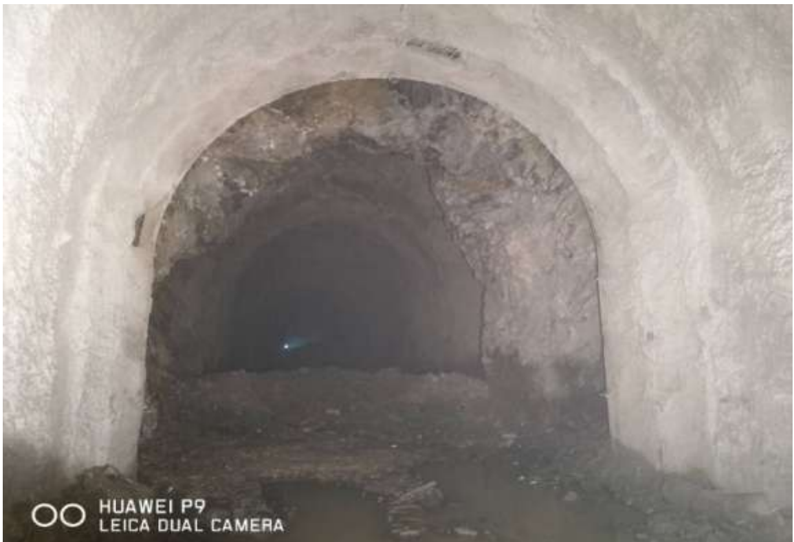
Break Through of HRT and Valve Chamber
