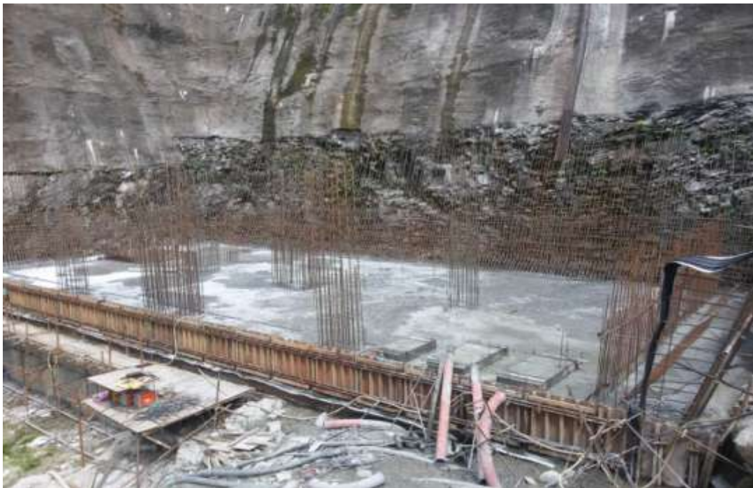
Raft Concrete work in auxiliary Powerhouse completed
