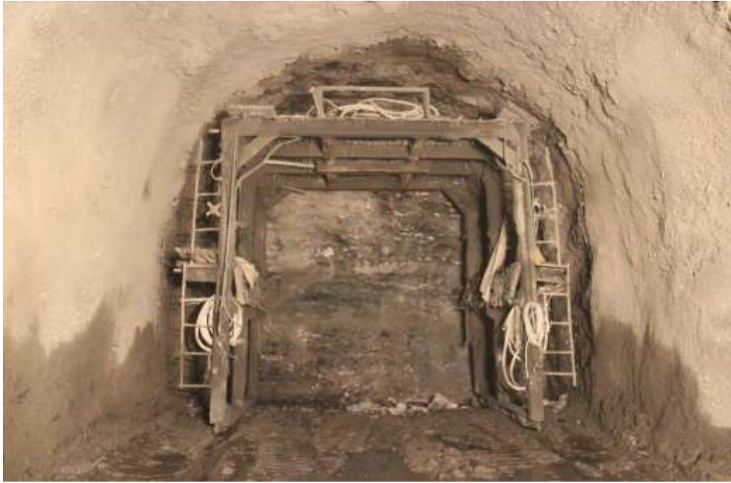
HRT Inlet -Tunnel face at chainage 698.5m
