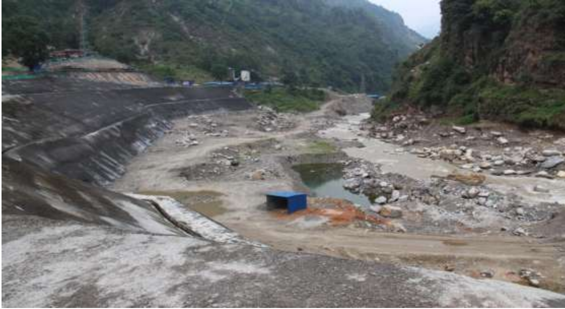
Headworks :Drilling and Jet grouting works of u/s coffer dam completed
