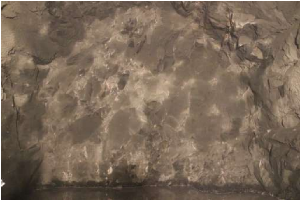
HRT Upstream from Adit 2-Tunnel face at chainage 4465.8m
