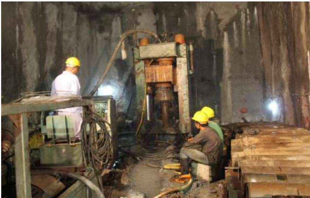
Pilot hole drilling at vertical pressure shaft in progress
