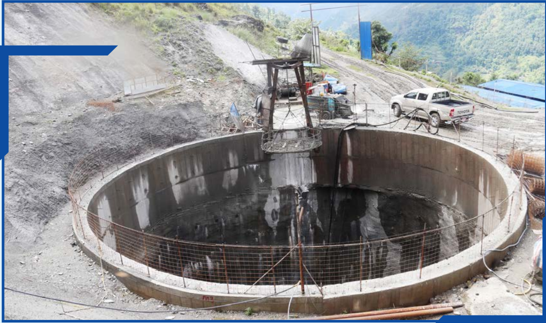
Surge Tank Excavation
