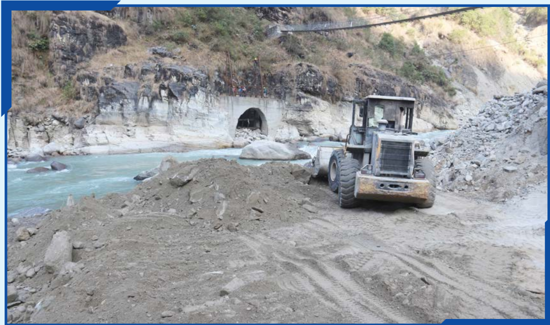
Cofferdam Construction
