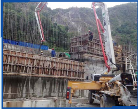
Concreting in Pier at Headworks
