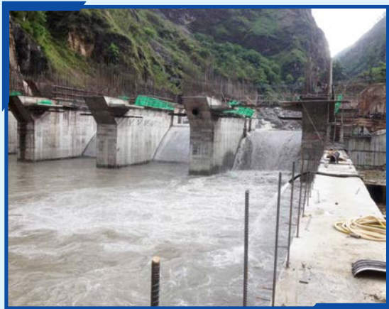
Completion of Spillway
