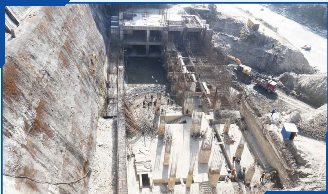
Cleaning Works at Powerhouse
