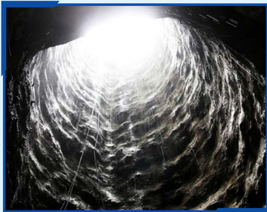
Completion of Surge Tank Excavation
