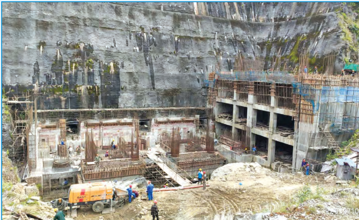
Construction Activities at Machine Hall & Auxiliary Powerhouse
