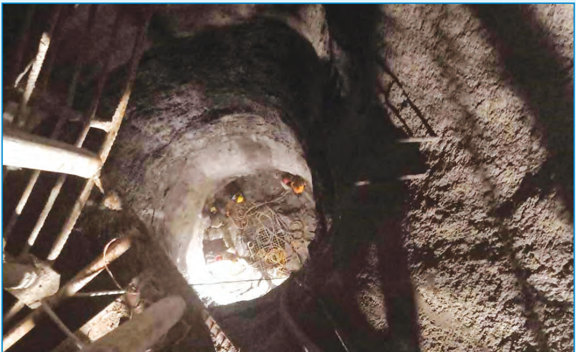
Vertical Penstock Shaft Widening Work
