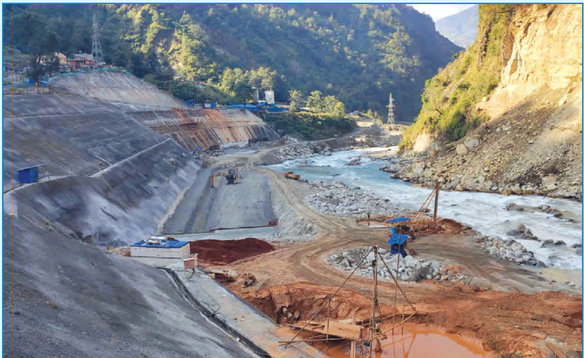
Bore Piling & Construction of Desilting Basin at Headwork
