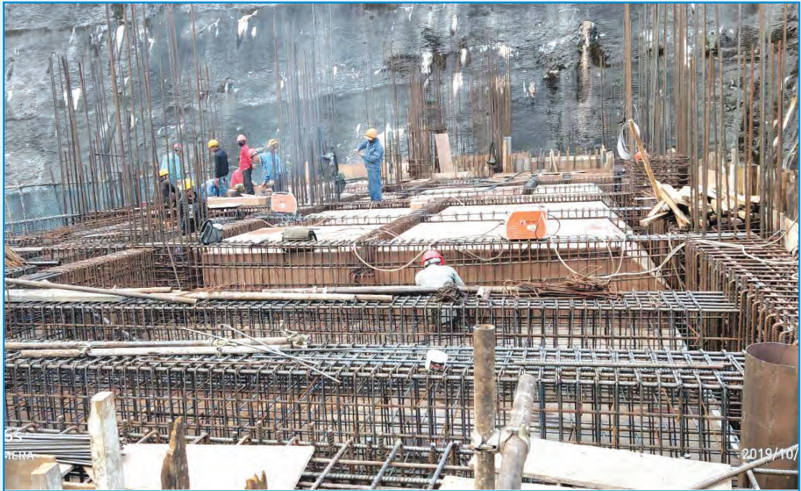
Construction Activities at Auxiliary Powerhouse
