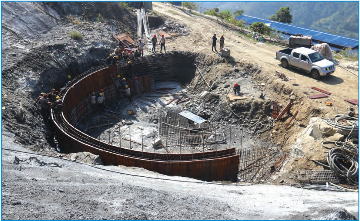
Widening of Surge Shaft Pilot Hole
