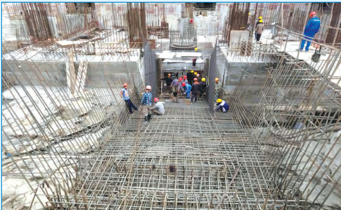
Construction Activities at Tailrace
