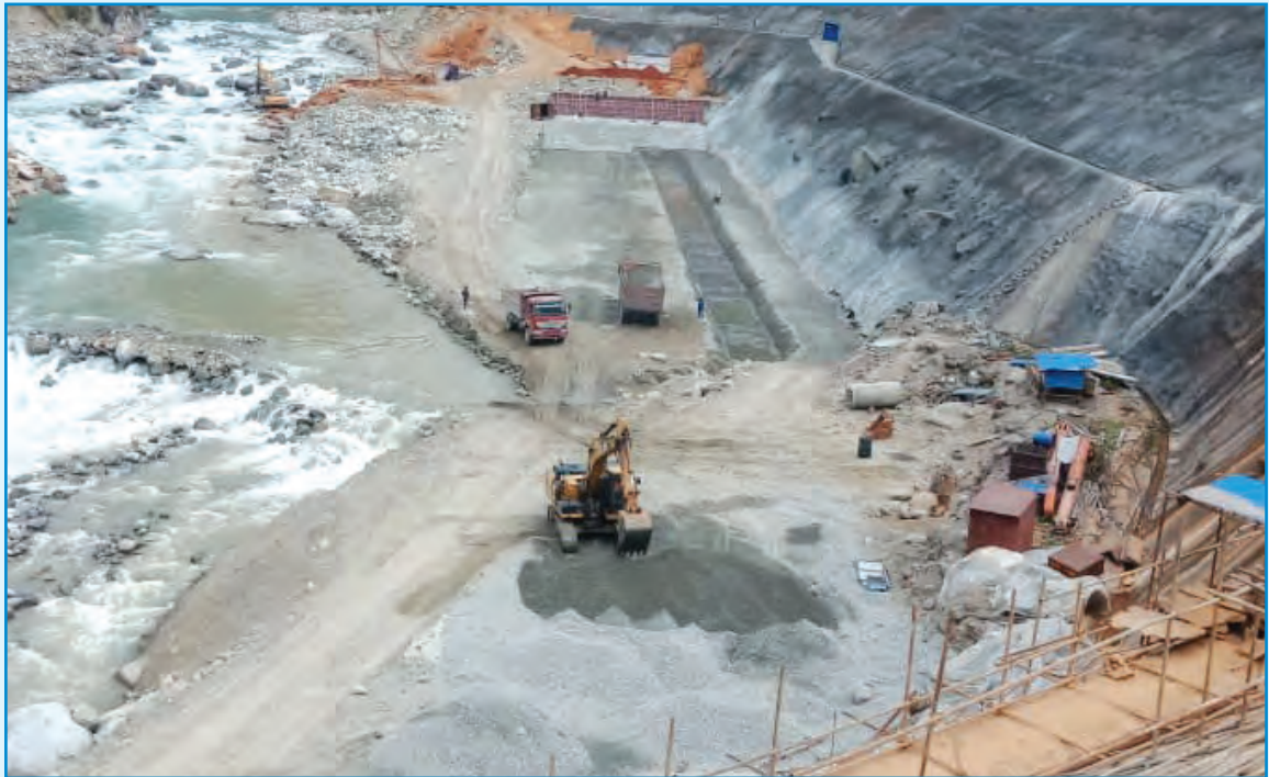
Construction Activities at Headwork
